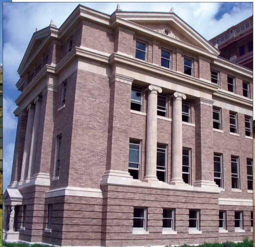
1914 Nueces County Courthouse
