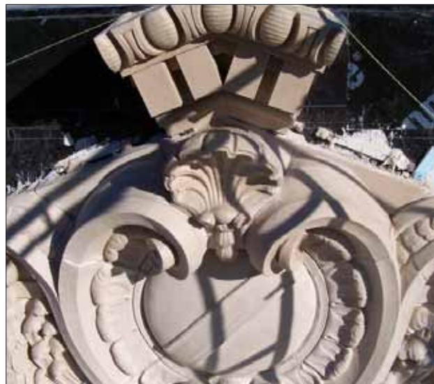
An 800-piece terra cotta jigsaw puzzle recreated the Williamson County Courthouse's original four ornamental porticos.
